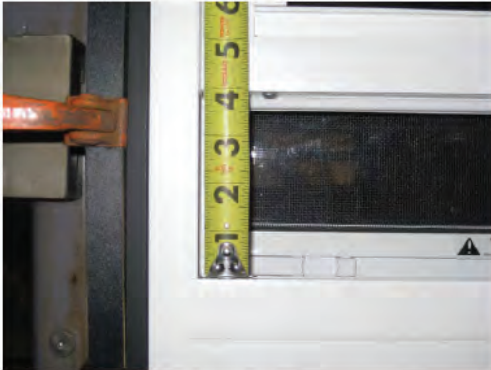
Photo No. 5 Window Opening Size Before Cycling
