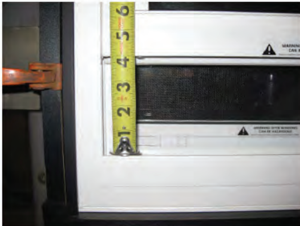
Photo No. 8 Window Opening Size after Cycling
