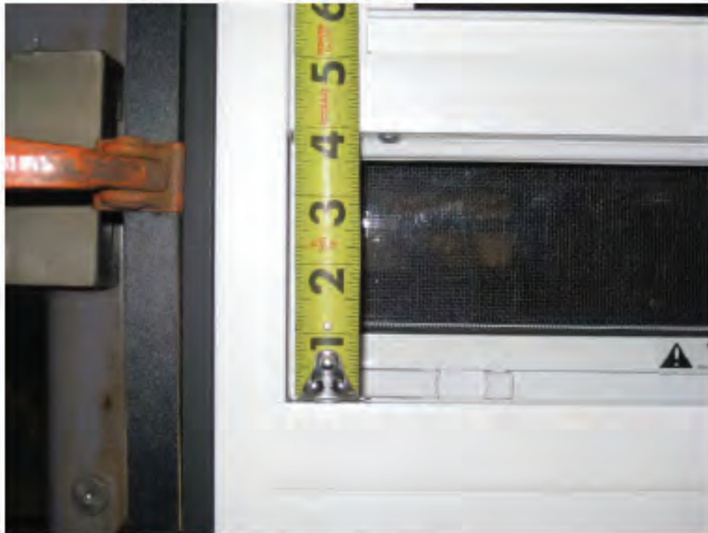
Photo No. 5 Window Opening Size Before Cycling
